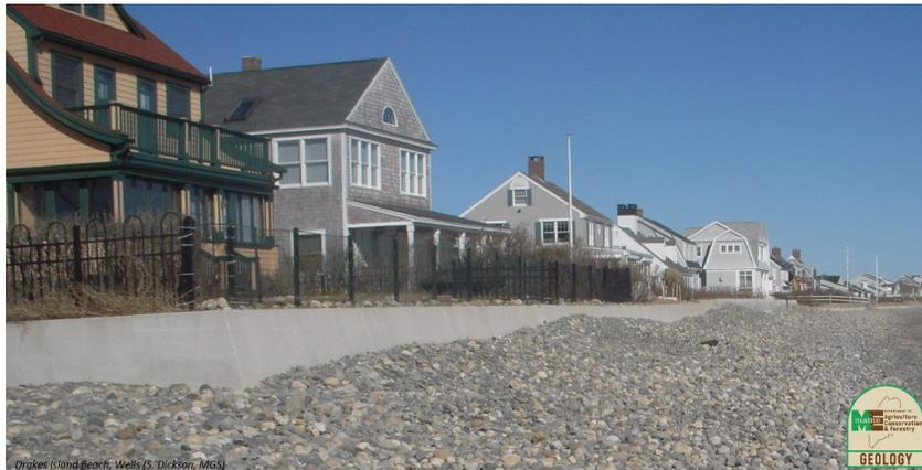
Figure A10. Cobble-trapping fences along Drakes Island Beach, Wells, ME.
