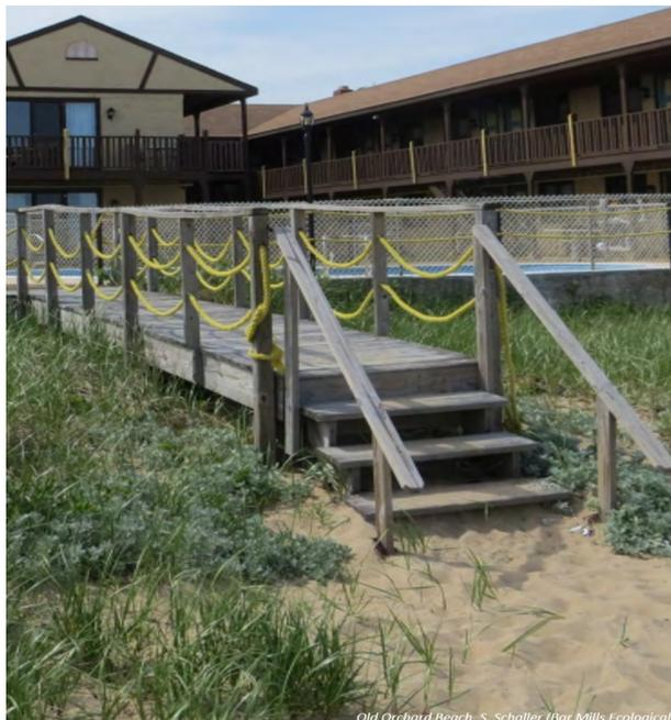
Figure A12. Example of a raised dune walkover from Old Orchard Beach, ME. Image from S. Schaller, Bar Mills Ecological.
