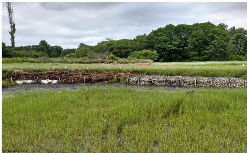
Figure C7. Example of a demonstration living shoreline treatment at an eroding marsh edge that utilizes aged oyster shell placed in coconut-fiber biodegradable bags (left side of image) and plastic-mesh gabion baskets (right side of image). The treatment also beneficially utilizes an in-place tree trunk as toe protection. Image by P. Slovinsky, MGS.
