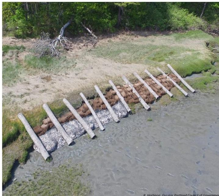
Figure B10. Example of a hybrid living shoreline at Maquoit Bay Conservation Lands, Brunswick, ME, along an eroding marsh edge which beneficially uses woody debris (logs) and integrates biodegradable bags and synthetic baskets filled with aged oyster shell. Image by R. Harbison, GPCOG.
