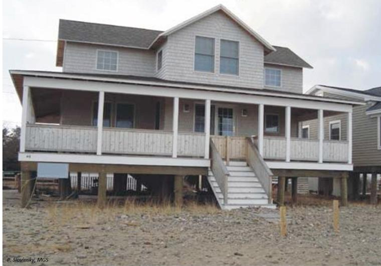
Figure C5. Example of a pile-supported foundation from a structure located in the front dune and within a flood zone. Image by P. Slovinsky, MGS.
