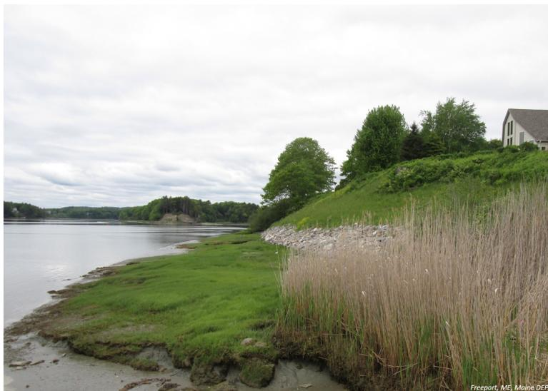
Figure B12. Example of bluff regrading, placement of toe armor, and planting with native vegetation from Freeport, ME. Image by Maine DEP.
